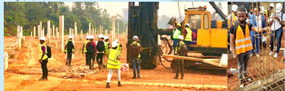
Field trip by Civil Engineering and Town Planning students
