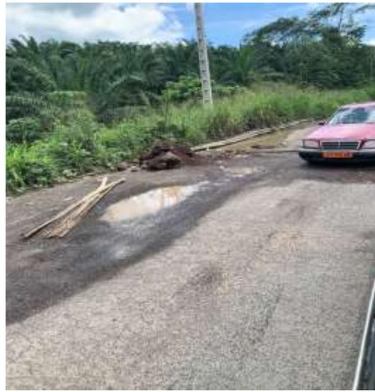
Figure 3. Rut and depression with worn out guardrails extending to the road lane at Mbanga entrance
